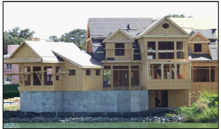
Construction continues (Photo by Ryan Mavity, Cape Gazette)
