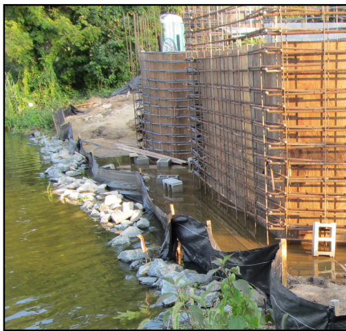
9’ concrete foundation arising from the lake
